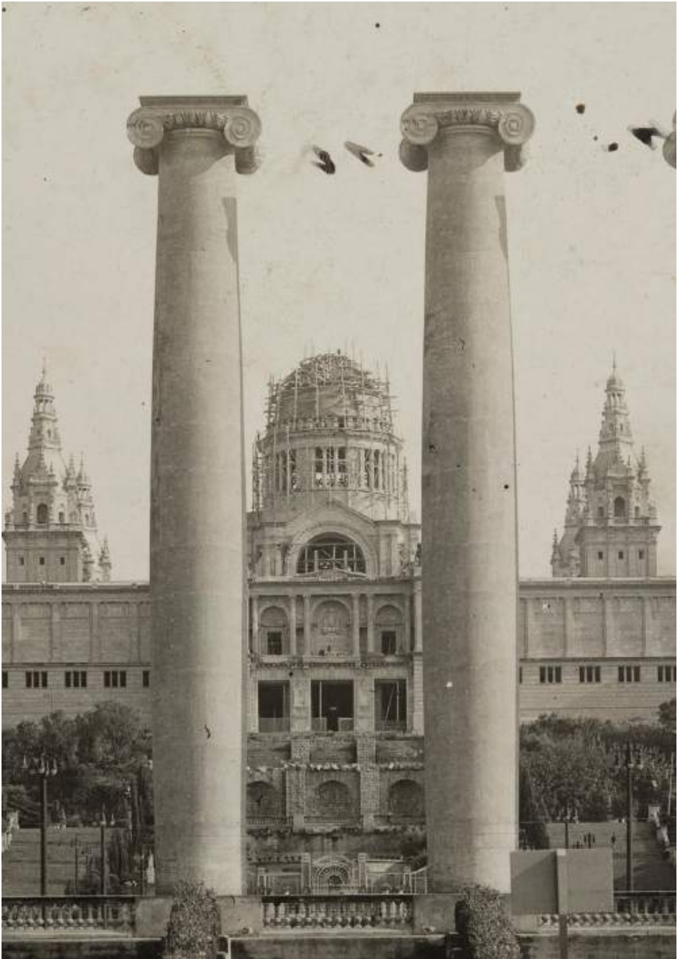
The Palau Nacional during construction.
