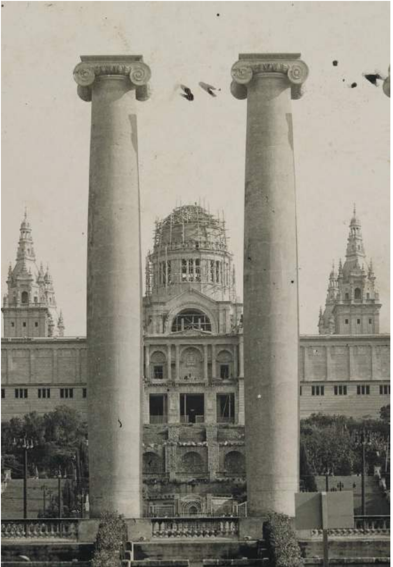
The Palau Nacional during construction.
